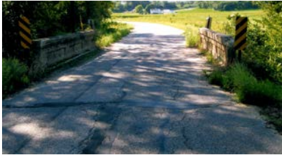
Skinner Road Bridge built in 1924
